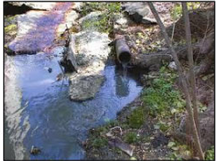
Figure 5: Illicit discharge (Source: EPA IDDE Manual: https://www3.epa.gov/npdes/pubs/idde_manualwithappendices.pdf )
